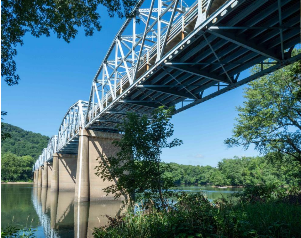
Highway 15 Bridge, Point of Rocks
