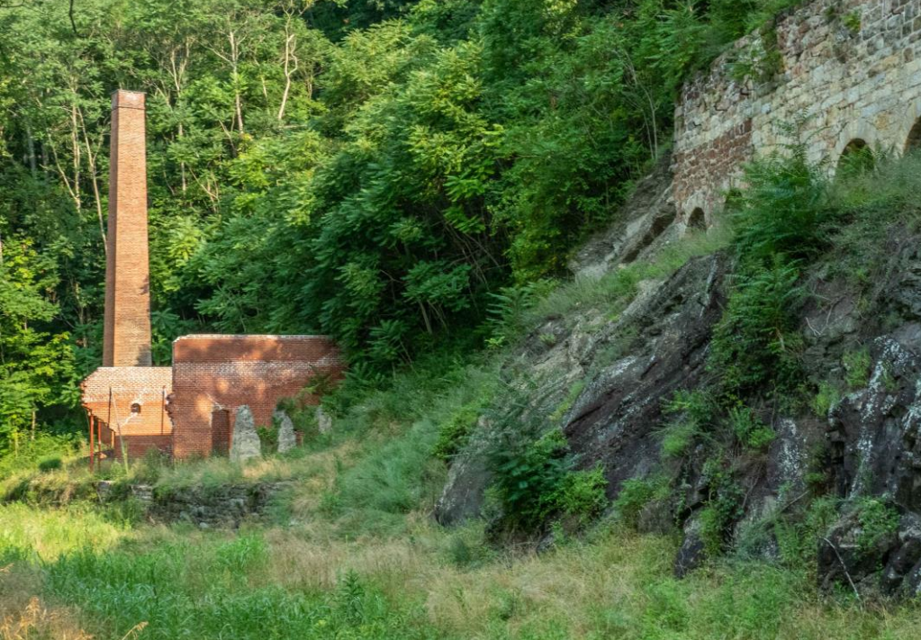
Round Top (limestone) Cement Mill Ruins - 8 kilns on right. 1838 – 1909. Put out of business by Portland cement.
