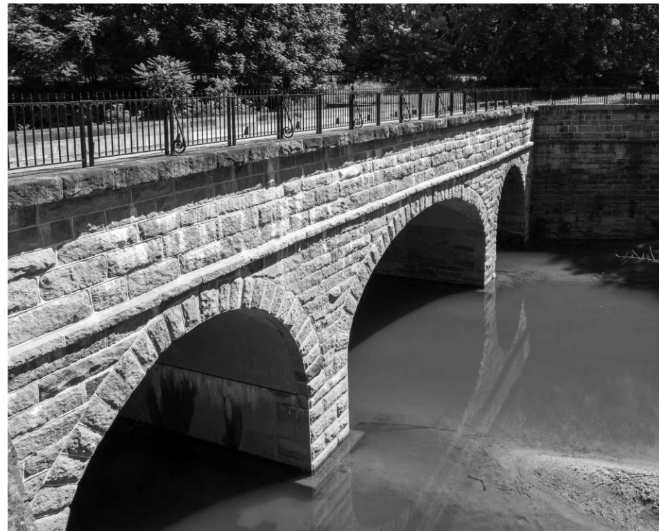
Catoctin Creek Aqueduct, north of Brunswick
