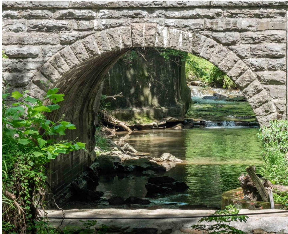
Railroad bridge, north of Brunswick
