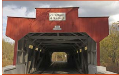
Stepped Portal of Geiger's Covered Bridge, Coriolana Simon
